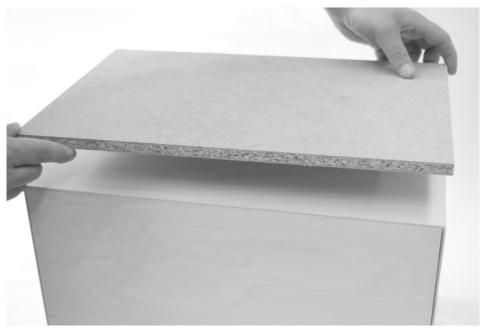
Put the pressure plate on the back panel, check the edges for flushness and press the pressure plate briefly.
