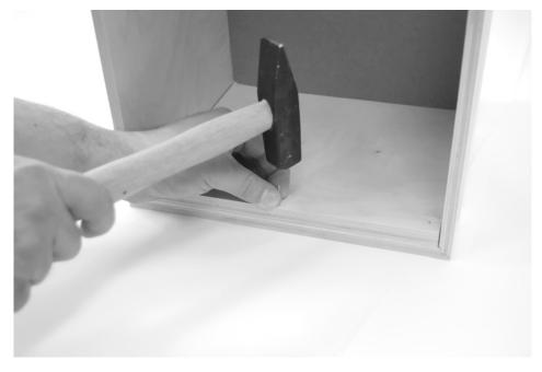
Fix the bottom strip with three nails in the pre-punched holes.
