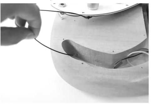
Pull the cable out of the hole far enough to ensure sufficient contact with the metallic surface when the bridge is installed. Earthing the strings reduces noise (humming).
